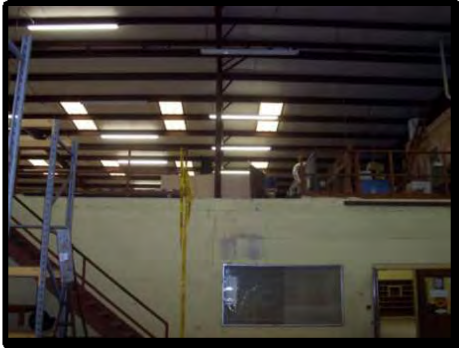
View of Mezzanine from ground floor
